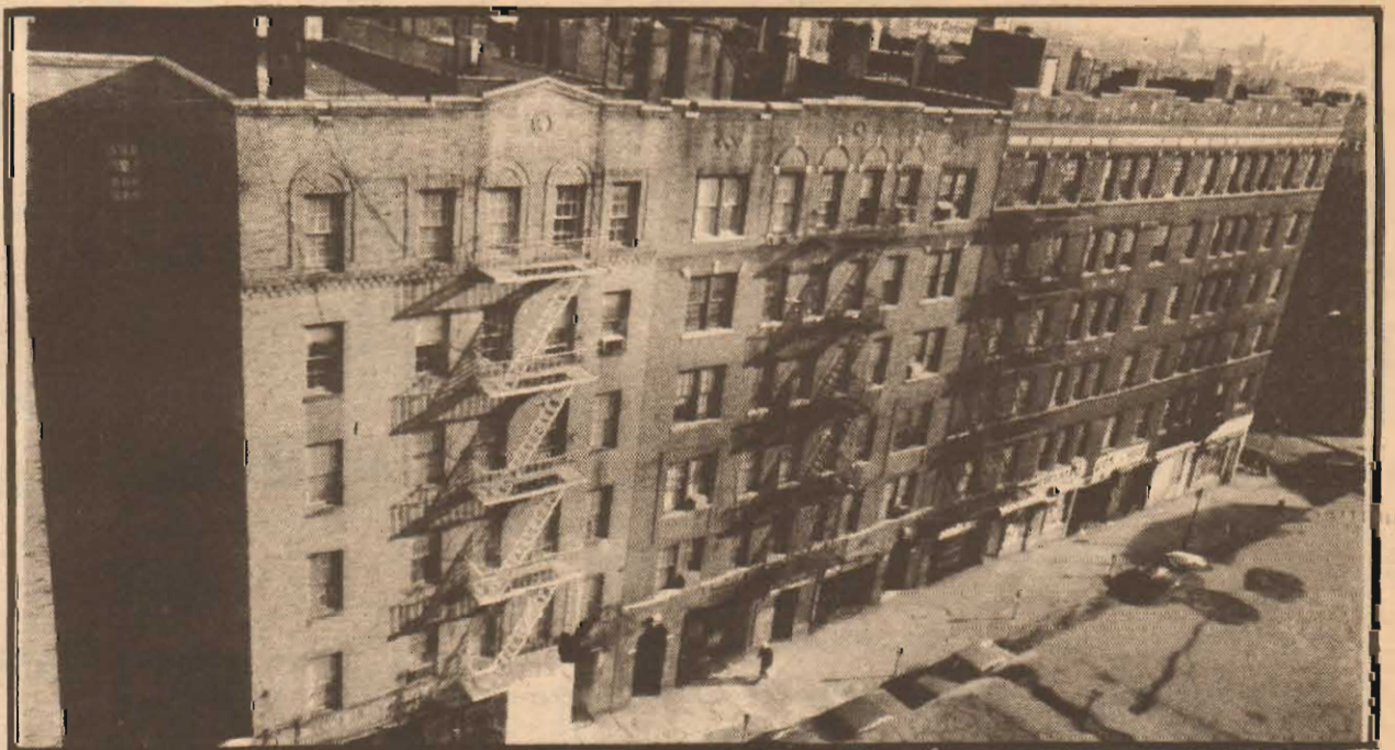
184th St. bet. Morris & Creston: Real estate speculators often set fires to drive out tenants and sell property at great profits. How else could you explain two deliberately set fires of the same type on the same block on the same night?
