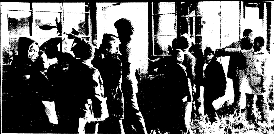
Children at Stella Wright Homes point to a few of many broken and boarded-up windows.
